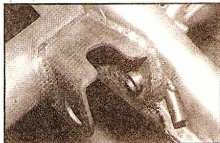
10-This is the finished product, as you can see Larry at Suspensions Unlimited did a beautiful job of welding the IRS pivots.
